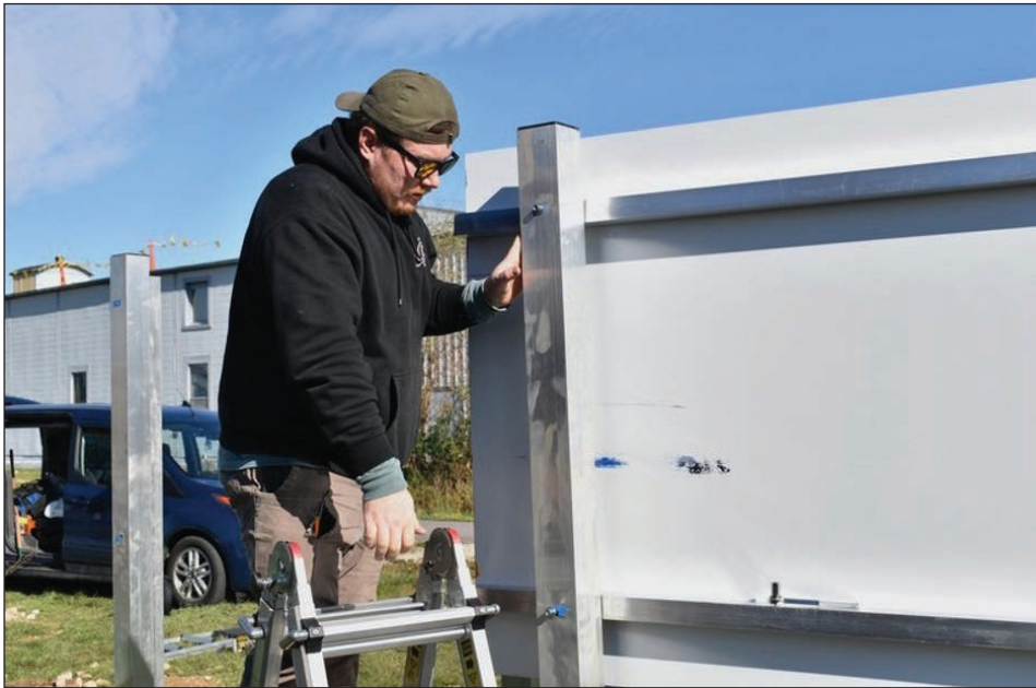
Chris' nephew Austin Azevedo helping install the first of 12 panels.
